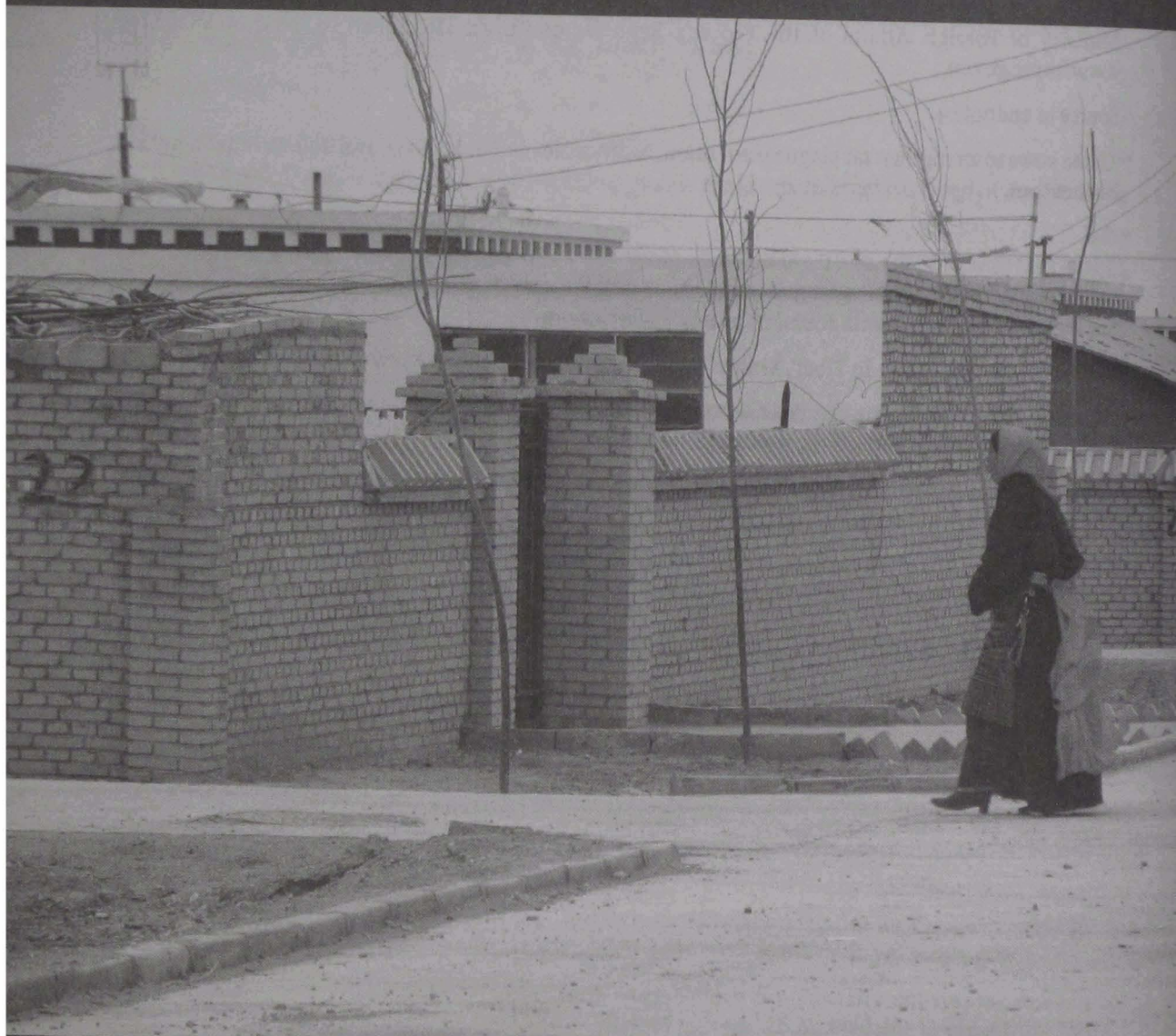
A building on the arid and sandy plains outside the southern areas of Golmud in Qinghai, at the beginning of the railway line to Lhasa. This Tibetan nomad settlement camp is one of the latest such projects completed in Tibetan areas. IMAGE: ICT.
